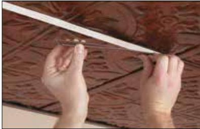
Applying GridMax Over T-bar Suspension Grid System
