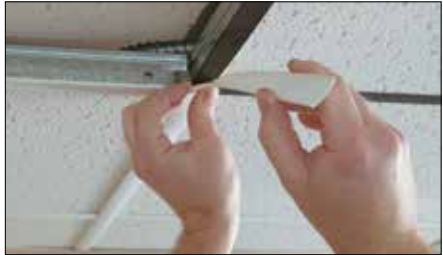
Applying GridMax Over T-bar Suspension Grid System
