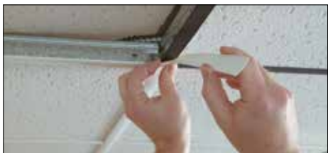
Applying GridMax over T-bar Suspension Grid System
