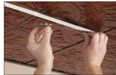
Applying GridMax Over T-bar Suspension Grid System
