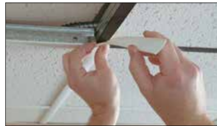
Applying GridMax Over T-bar Suspension Grid System
