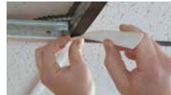
Applying GridMax Over T-bar Suspension Grid System
