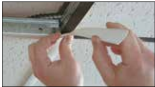
Applying Gridmax over T-bar suspension grid system
