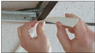
Applying Gridmax over T-bar suspension grid system
