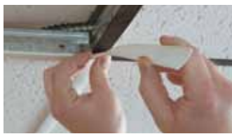
APPLYING GRIDMAX OVER T-BAR SUSPENSION GRID SYSTEM
